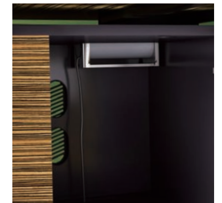
柜体内部走线，既美观，又隐蔽。 wiring inside the cabinet body is concealed and beautiful.
